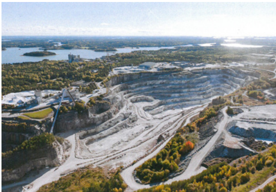
Kalstensbrottet (foto: Nordkalk)
